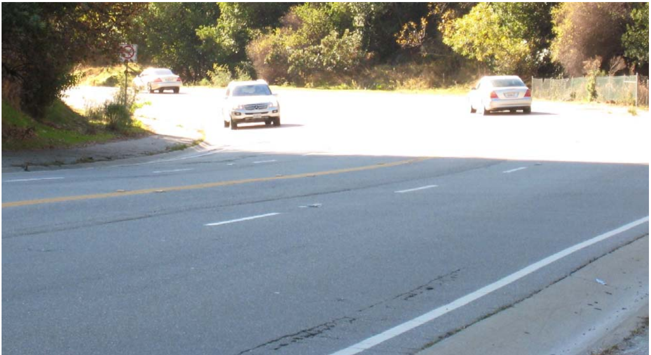
Figure 1: A part of Palisades Drive canyon section, with 4 lanes, sidewalk, and gutter showing
